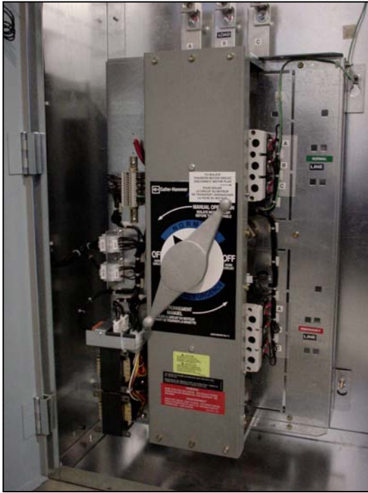
Figure 3 - Typical Power Panel for 200-1200A models
